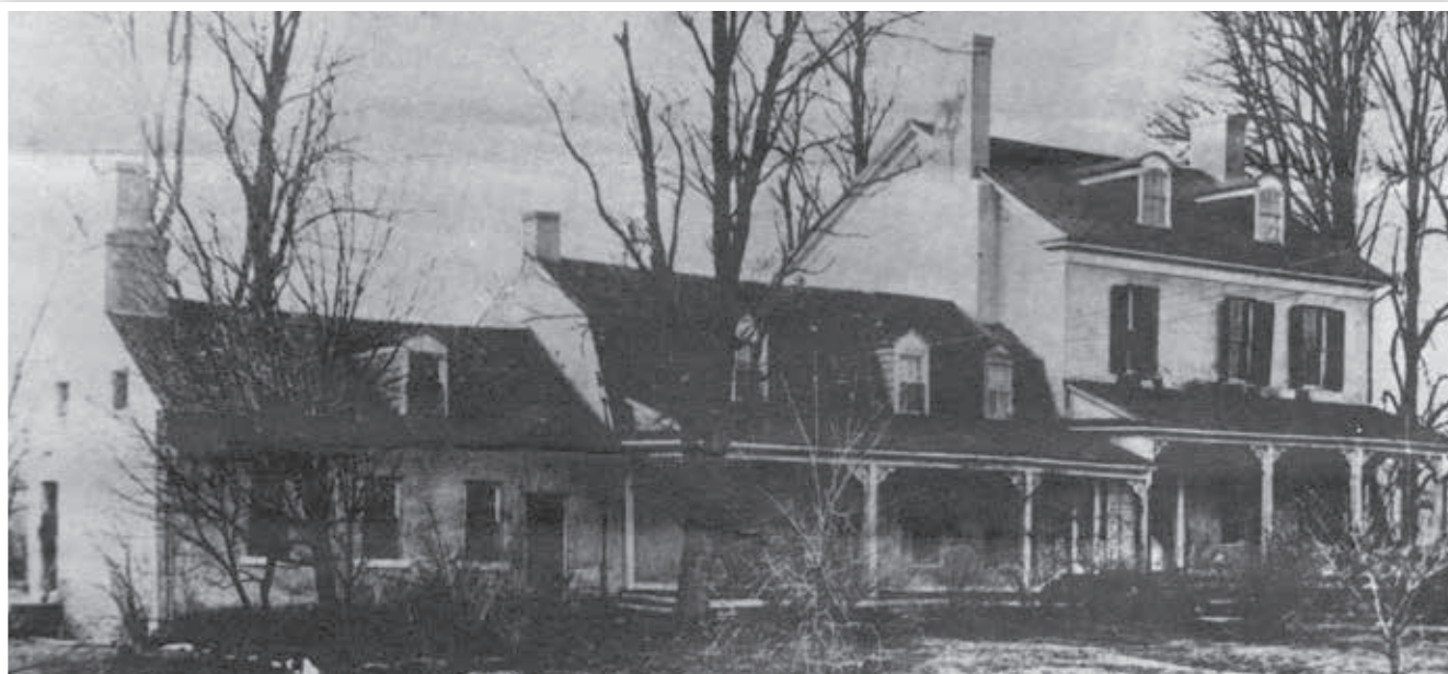
Spyglass houses, similar to the Hereford House, are found throughout the Northeast. This type of house is made when sections are continually added to an original house.
