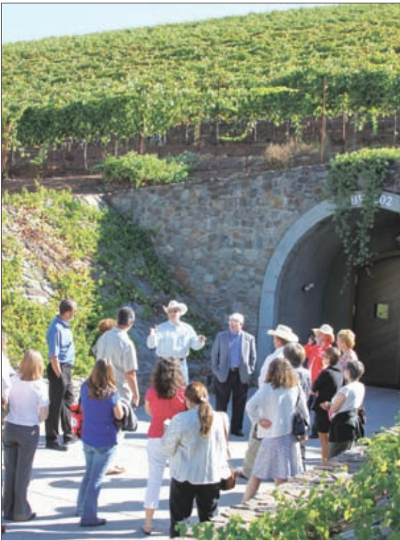
A highlight of the tour was going into the caves where the Kunde family wine ages. The caves are built deep into the hillside behind the winery and include more than 32,000 square feet of tunnels.
