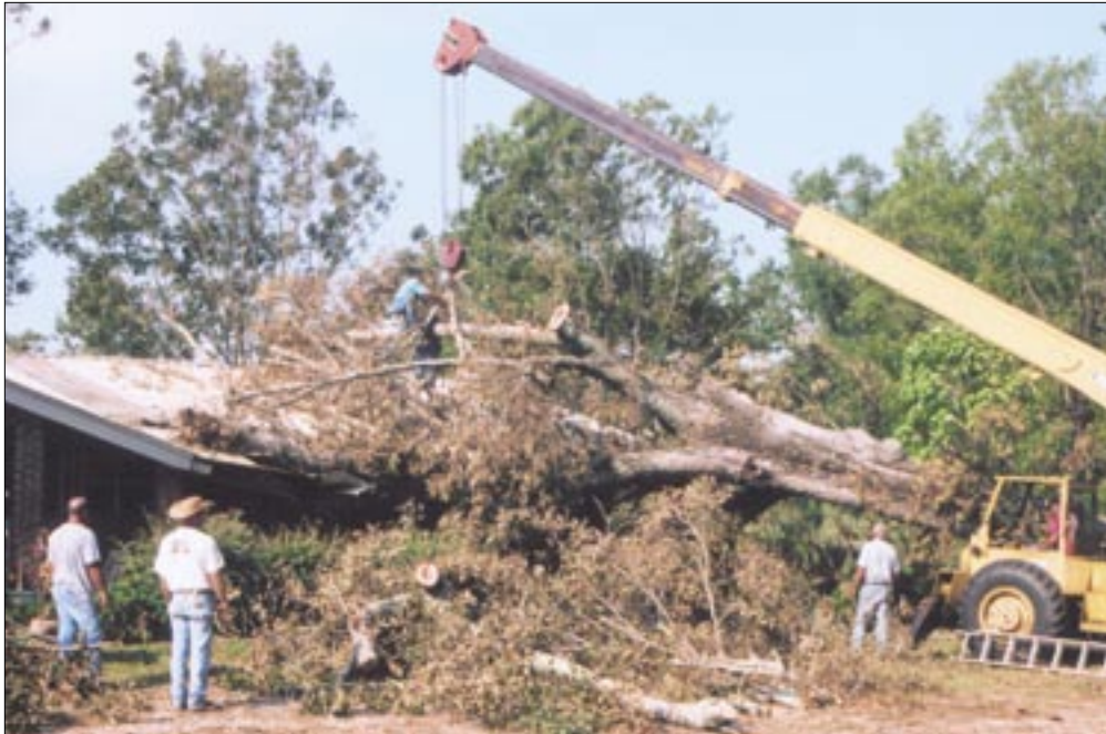
Hurricane Katrina knocked a 52-inch live oak tree onto the home of Halton and Jean Herring of Punkin Ridge Farm, Beaumont, Miss.
